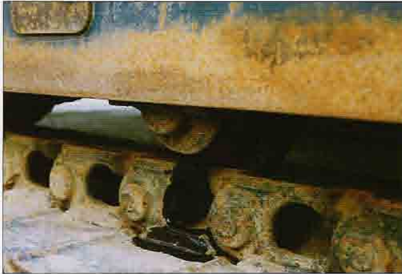
Oil leakage out of track roller
